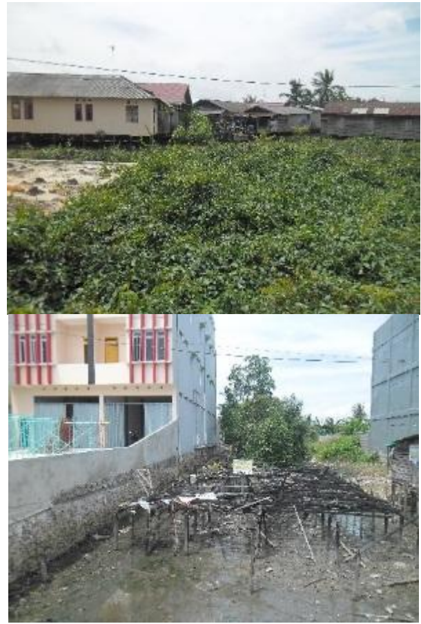
Figure 13. Conversion mangrove and swamp area become housing area RT.42 and shopping area on Jl. Mulawarman.
