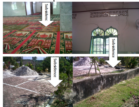
Gambar 2. Foto Fenomena Subsidence
