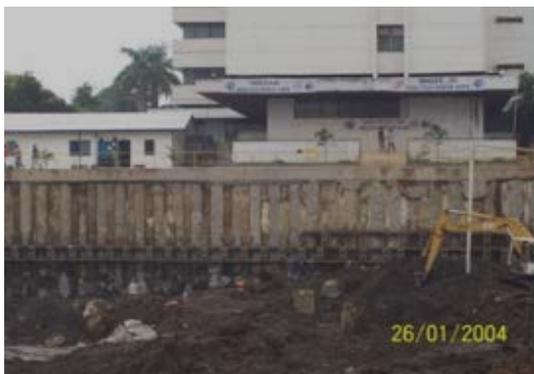
Gambar 3. *Cement Bentonite Pile*
