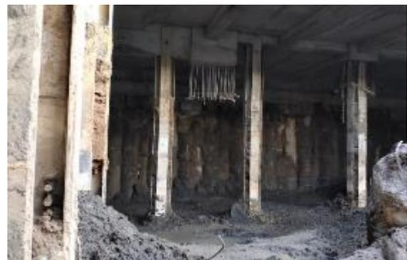
Gambar 5. *Secant Pile & Kingpost*
