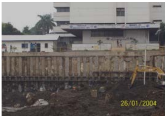
Gambar 3. Cement Bentonite Pile
