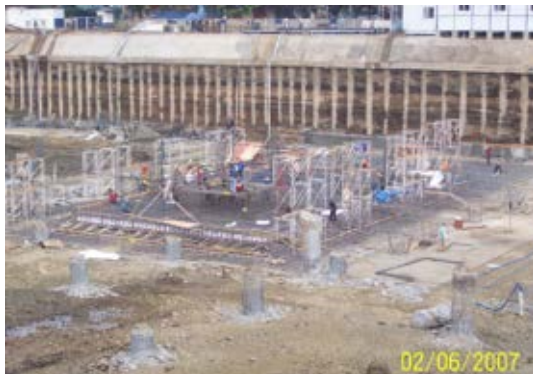
Gambar 2. Soldier Pile (Tiang Bor)
