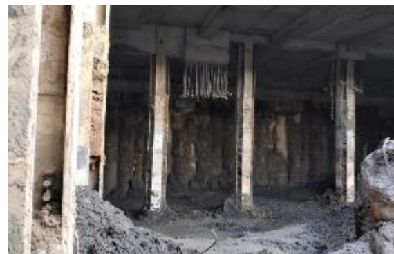
Gambar 5. Secant Pile & Kingpost
