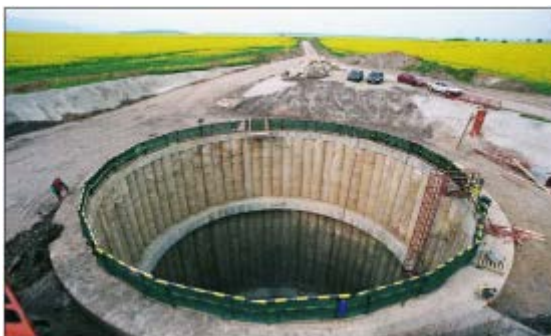
Gambar 4. Secant Pile
